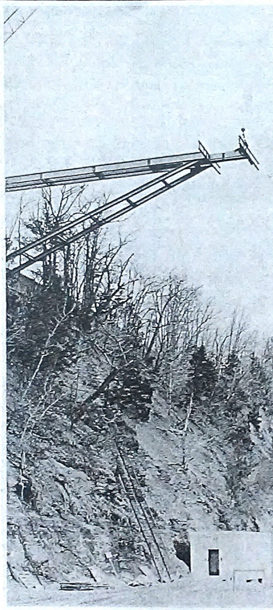
A VERTICAL GONDOLA is being constructed at the Bristol Harbor Village development at Seneca Point on Canandaigua Lake. Two enclosed cars, each seating four persons, will hang from cables attached to the steel structure in the upper portion of the photos. Purpose of the facility is to provide easy access to the development's private beach and dock. Photo at left shows stairs now used to reach the beach. At right, the approximate 120-foot drop is shown from balcony of one of the housing units. (Messenger photos)
