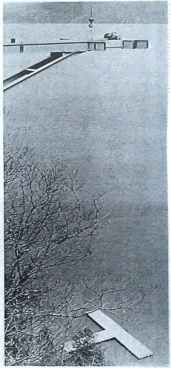
A VERTICAL GONDOLA is being constructed at the Bristol Harbor Village development at Seneca Point on Canandaigua Lake. Two enclosed cars, each seating four persons, will hang from cables attached to the steel structure in the upper portion of the photos. Purpose of the facility is to provide easy access to the development's private beach and dock. Photo at left shows stairs now used to reach the beach. At right, the approximate 120-foot drop is shown from balcony of one of the housing units. (Messenger photos)
